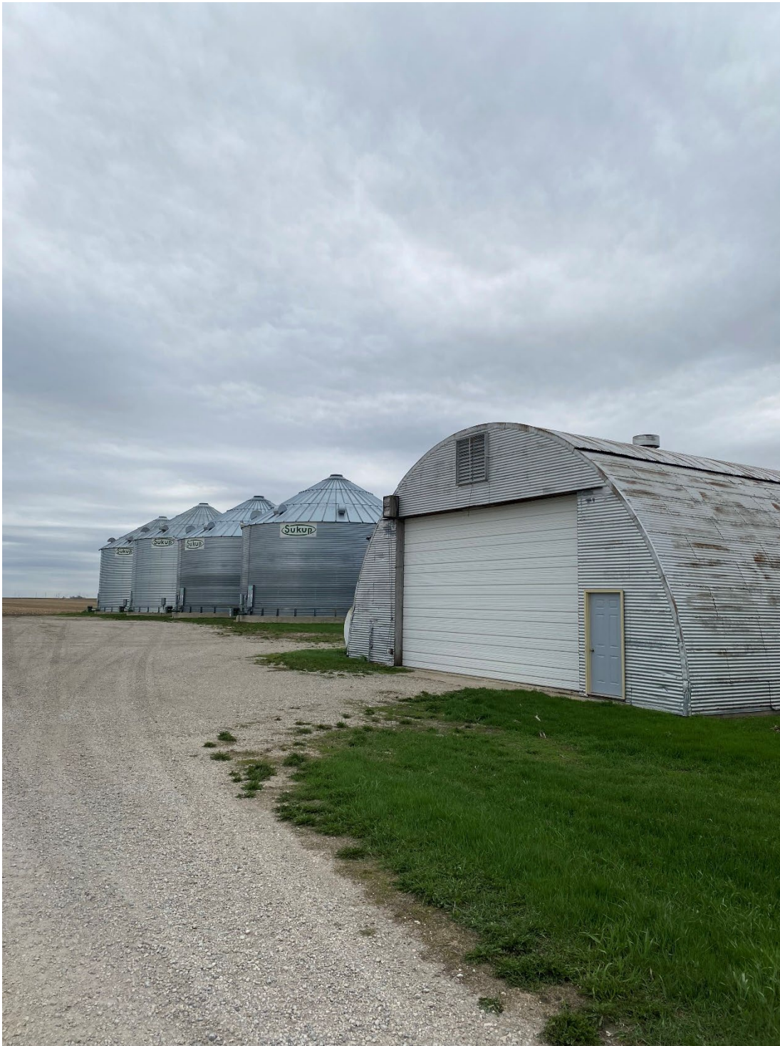
Quonset shed and 48 foot bins looking South The smaller bins are between the shed and large bins
