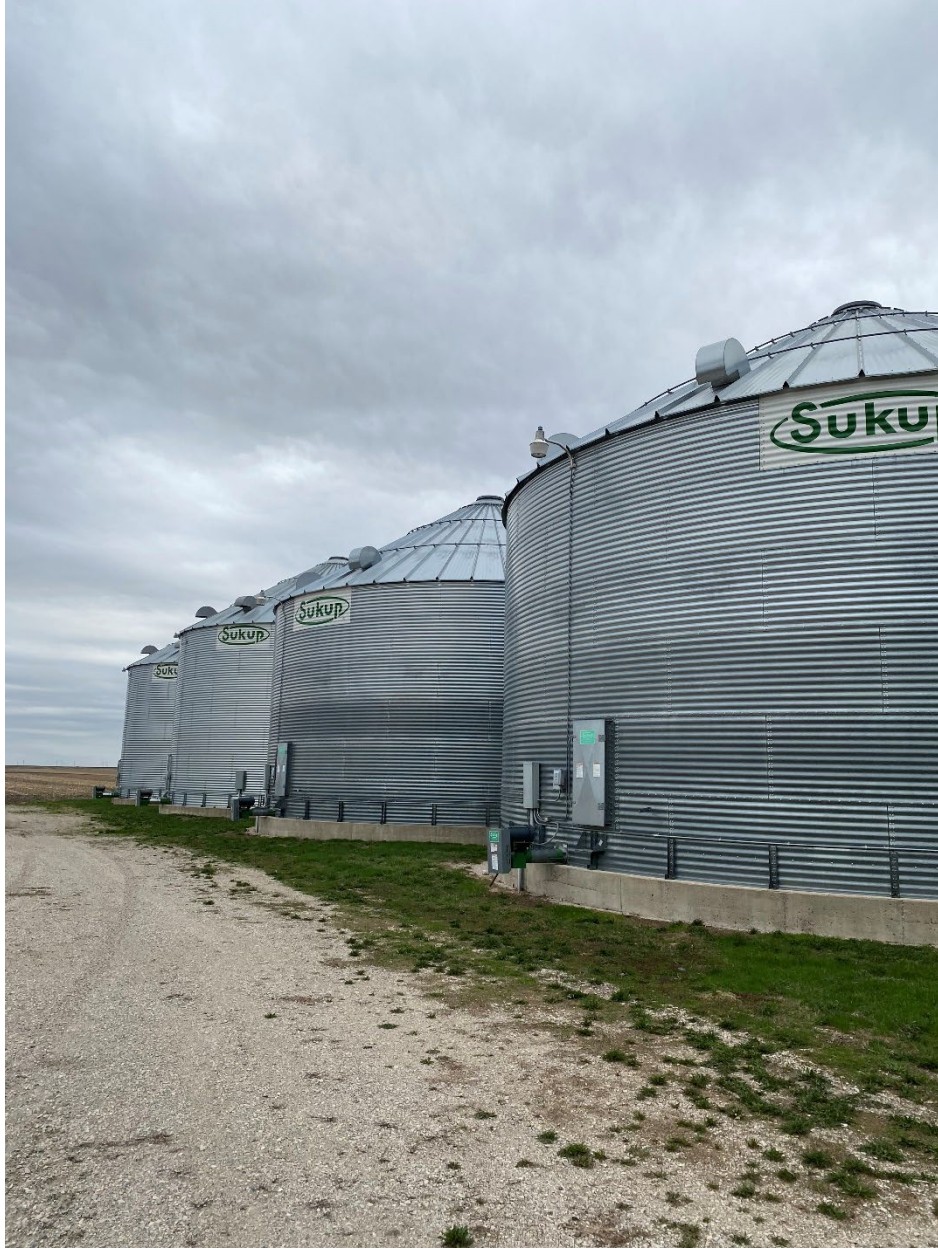
48 Foot Bins Looking South
